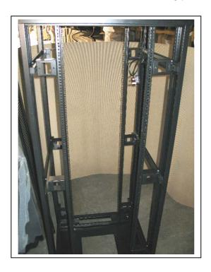
Carefully install the front and rear vertical profiles (x4 in total, x2 per side) on the installed 'Box Spacers'.
