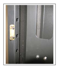
Locate the supplied 'Door Stoppers (x4 supplied on smaller Cabinets, x8 on taller Cabinets). The brass-coloured right angled small brackets should be screwed via 2 screws half-way up on the front/rear facing facets of the frames (locate the holes for these beforehand).
