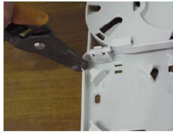
Pic7: right-routing leads in box entrance
