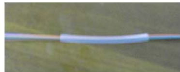
Pic5: use EVA transparent tube to protect the stripped fiber
